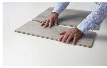
To disengage on the short side, slide the planks the opposite direction
